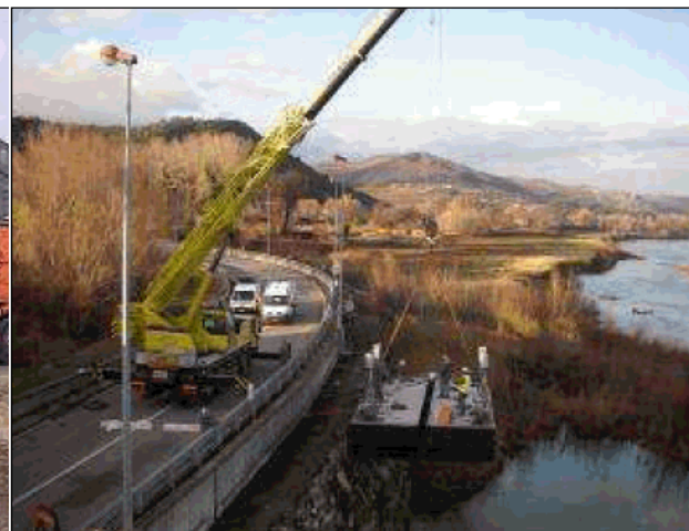
Figure 79 –Atelier de forage
